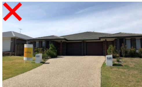
Dark materials and roof (source: Arkhefield)
