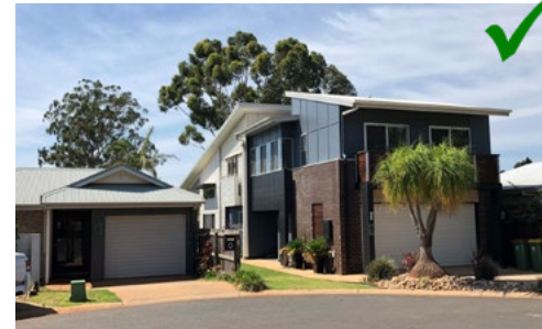
Appropriate setback between single storey and two storey dwellings to provide better daylight access, improves privacy and allows zone for landscape. (source: Arkhefield)
