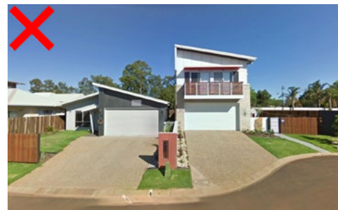
Two storey dwelling has zero setback to adjoining single storey dwelling and is not sympathetic in scale (source: Arkhefield)
