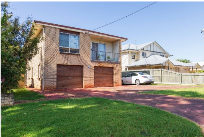
Image 21: Two-storey brick and timber clad homes with garages to the street and no front fence
