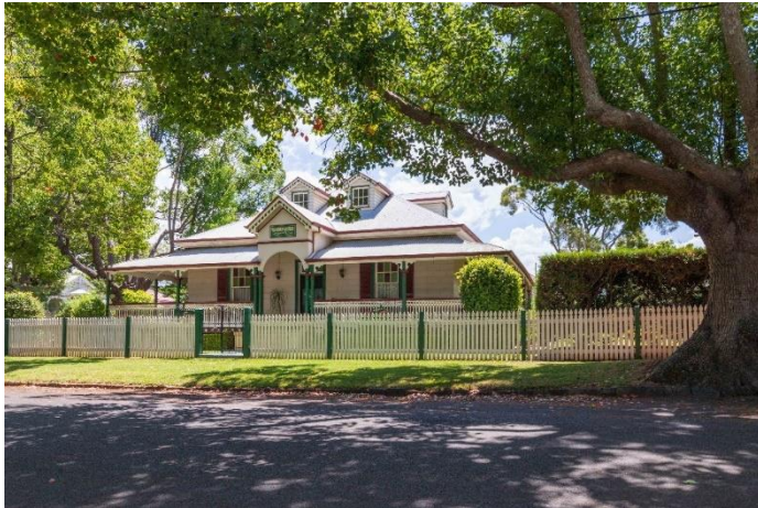
Image 7: Stately homesteads on large lots with significant trees and heritage kerbs
