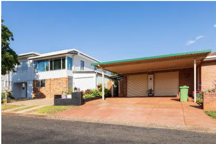
Image 14: 2-storey dwelling and brick home with wide driveway and double garage
